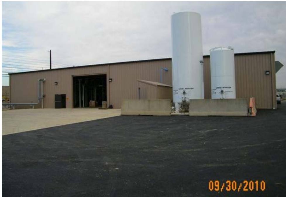
Figure A.108. X-675 Plant Nitrogen Station
