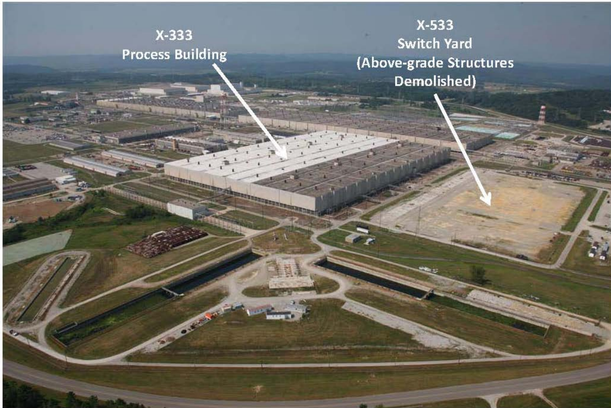
Figure A.102. X-533 Switchyard
