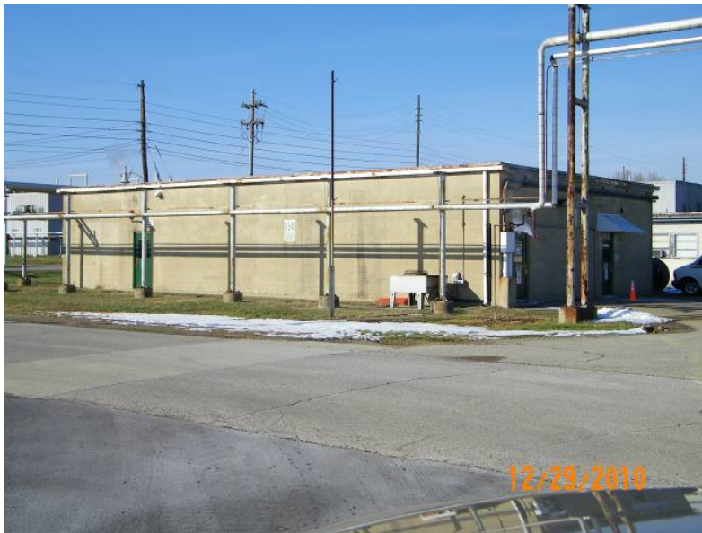
Figure A.64. X-540 Telephone Building
