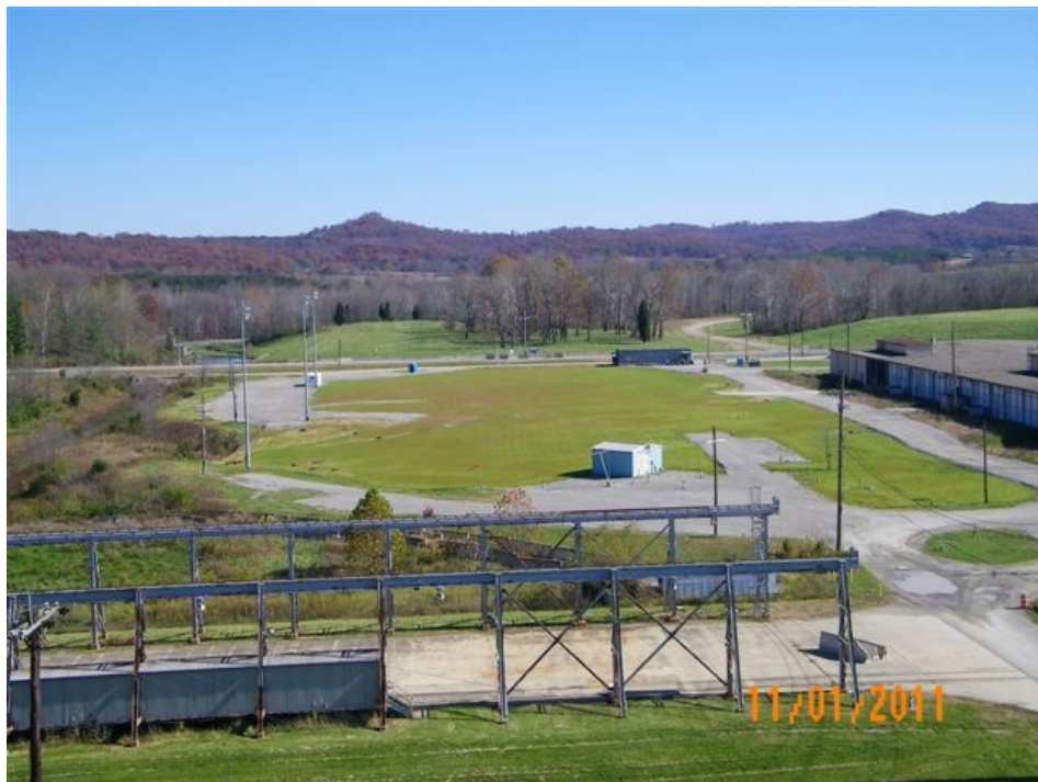
Figure A.143. X-747G Precious Metal Scrap Yard following IRM
