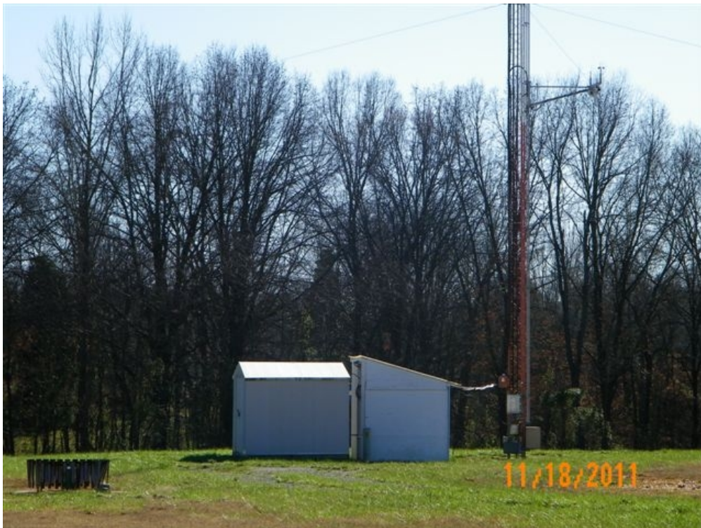
Figure A.152. X-120H Sheds
