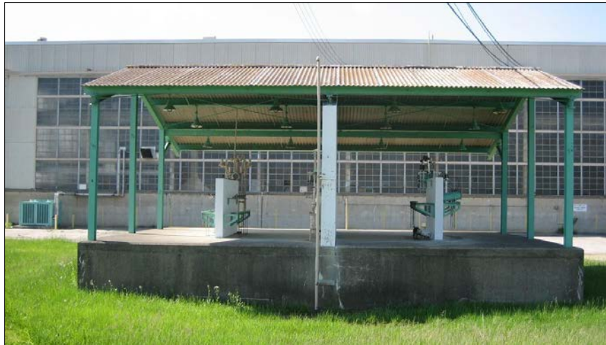
Figure A.39. X-720A Maintenance & Stores Gas Manifold Shed Prior to Demolition
