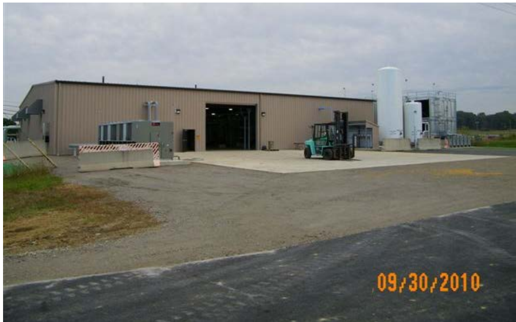
Figure A.109. X-670 Dry Air Plant
