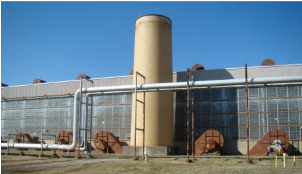
Figure A.20. X-700 Converter Shop & Cleaning Building
