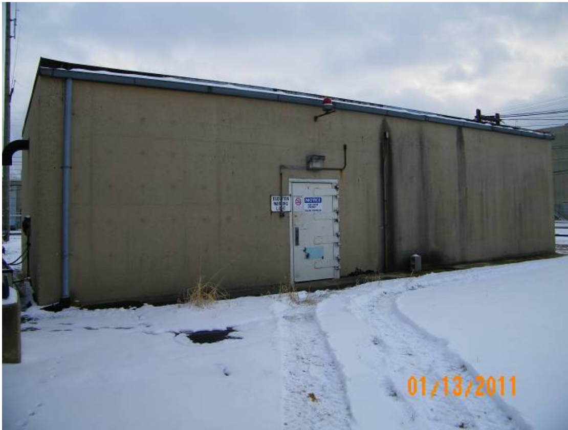
Figure A.60. X-300A Process Monitoring Building
