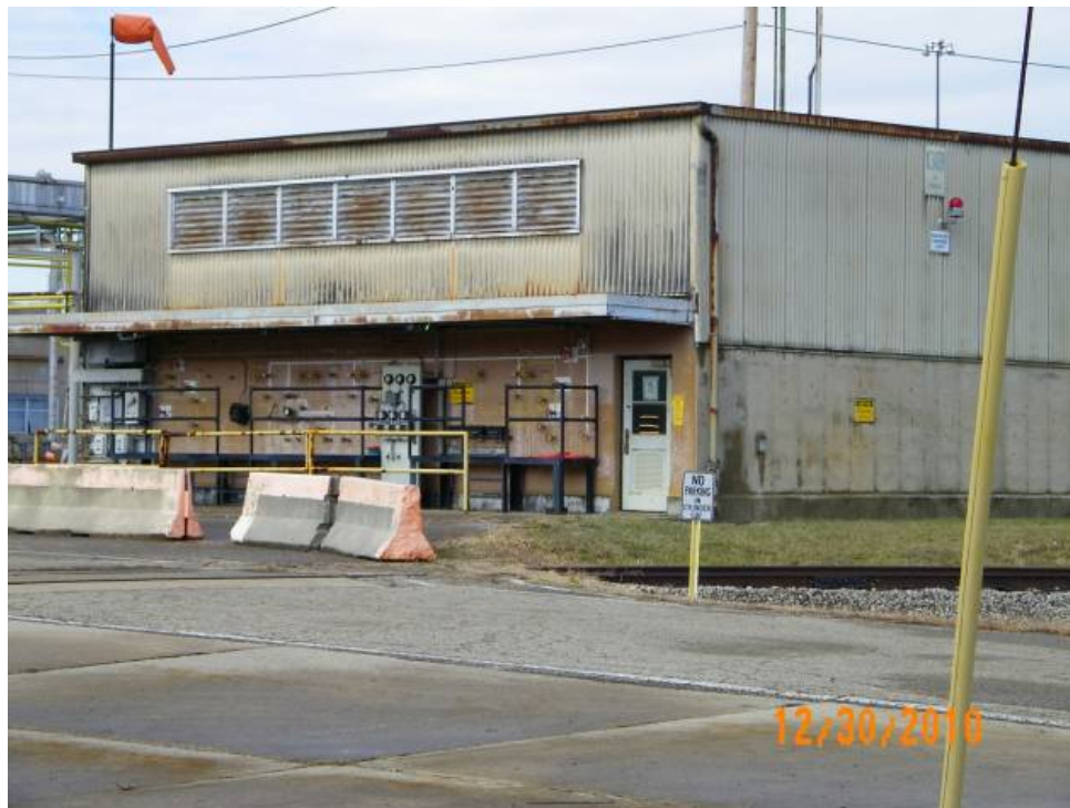
Figure A.17. X-342B Fluorine Storage Building
