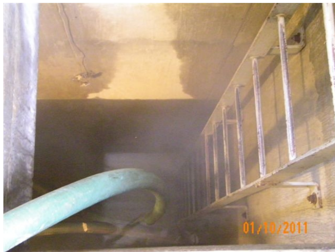
Figure A.27. X-705D Heat Booster Pump Building
