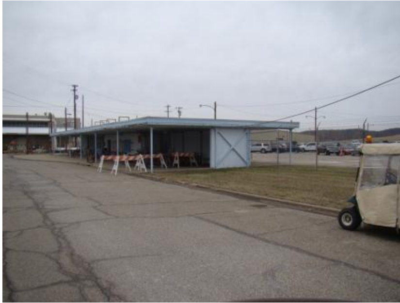
Figure A.45. X-108B North Portal and Shelter
