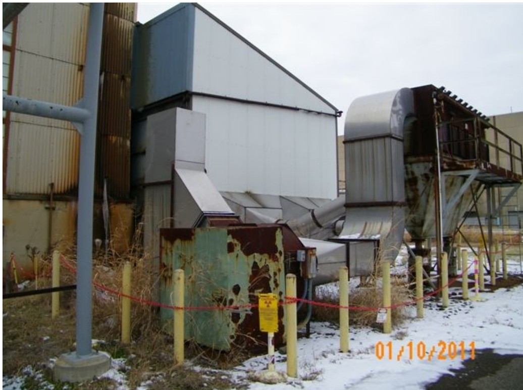
Figure A.21. X-700B Sandblast Facility and Observation Booth
