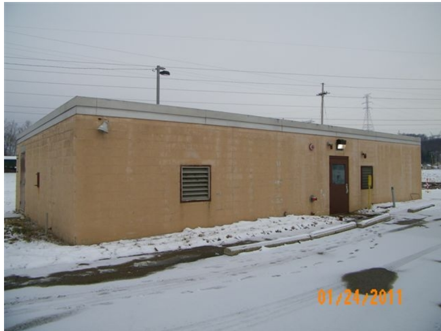
Figure A.99. X-6619 Sewage Treatment Plant, Filter and Chlorine Building
