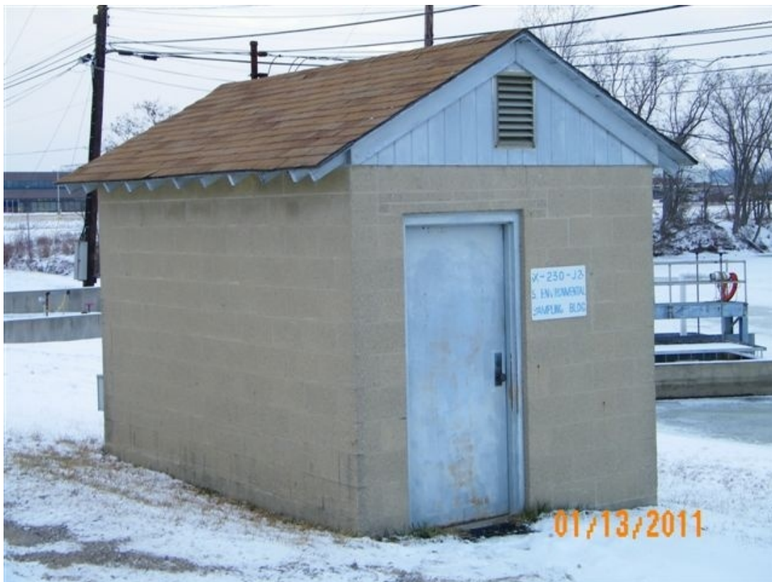
Figure A.153. X-230J2 South Environmental Sample Station
