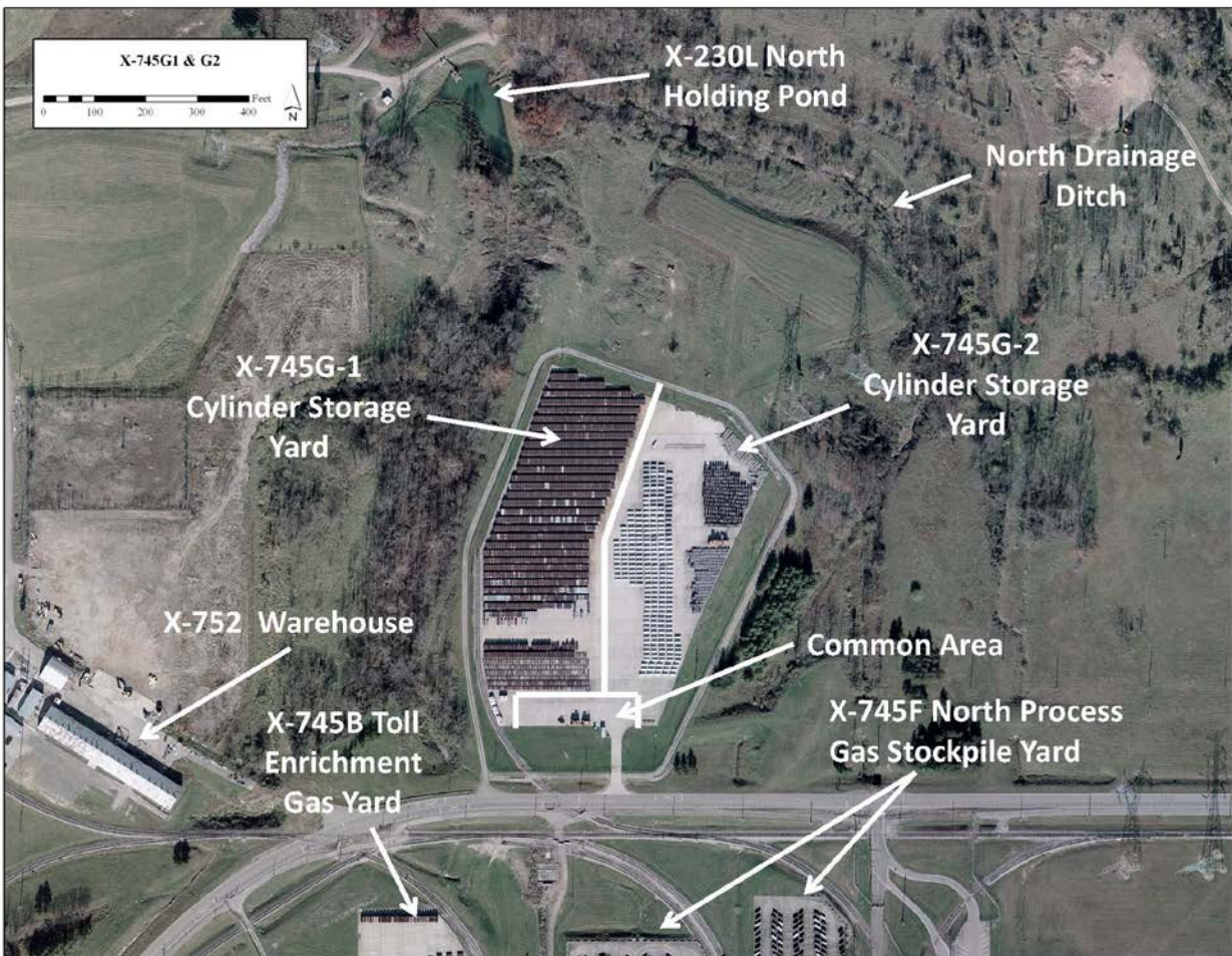
Figure A.135. X-745G-2 Cylinder Storage Yard (2006-2007 Aerial Photography)
