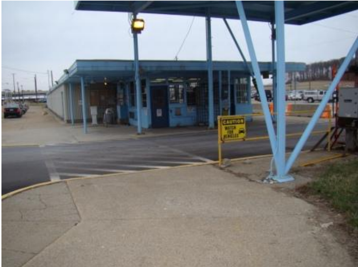
Figure A.44. X-108A South Portal
