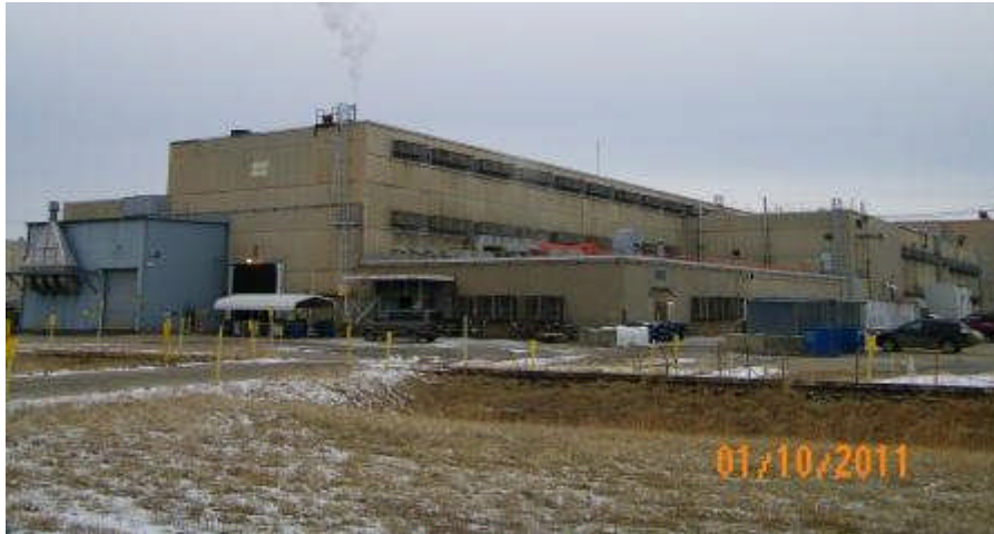
Figure 4.7. X-705 Decontamination Building at PORTS
