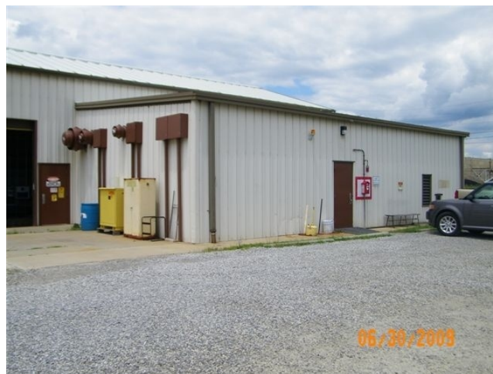
Figure A.173. X-622 South Groundwater Treatment Facility Exterior
