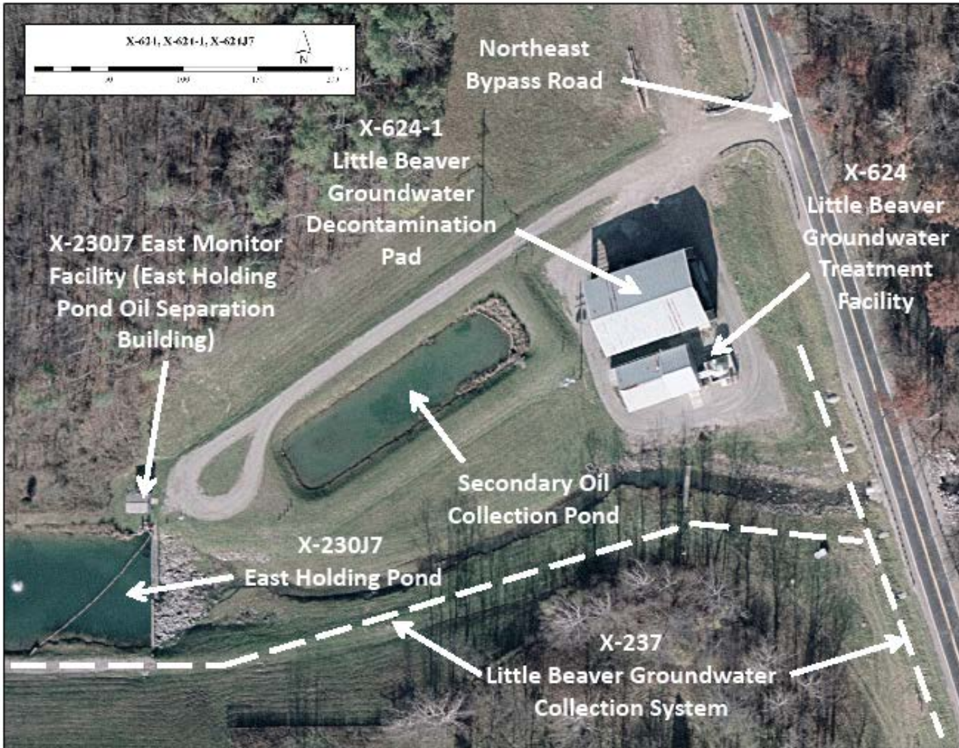
Figure A.176. X-237 Little Beaver Groundwater Collection System and X-624 Little Beaver Groundwater Treatment Facility (2006-2007 Aerial Photography)
