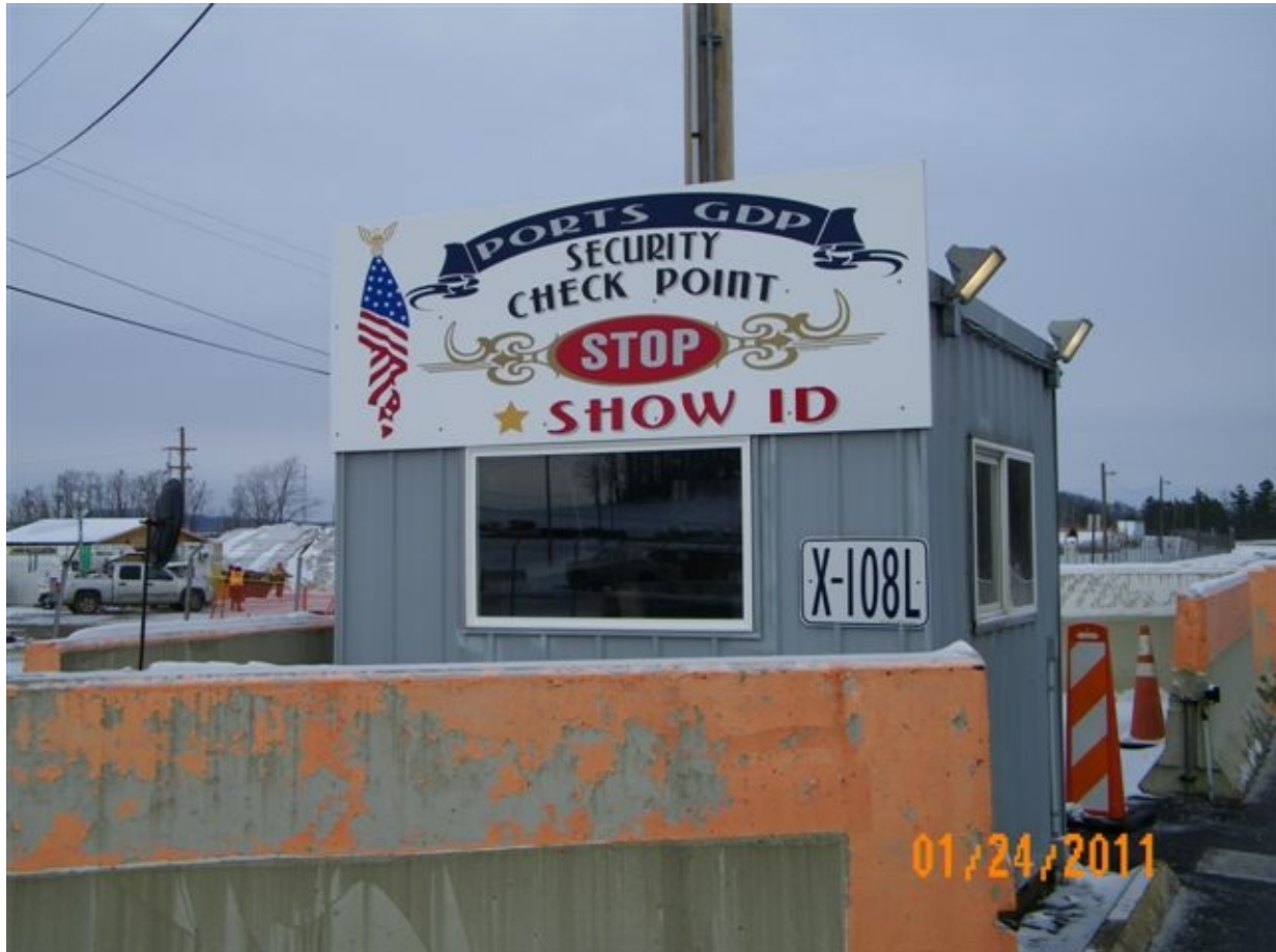
Figure A.49. X-108L East Security Portal
