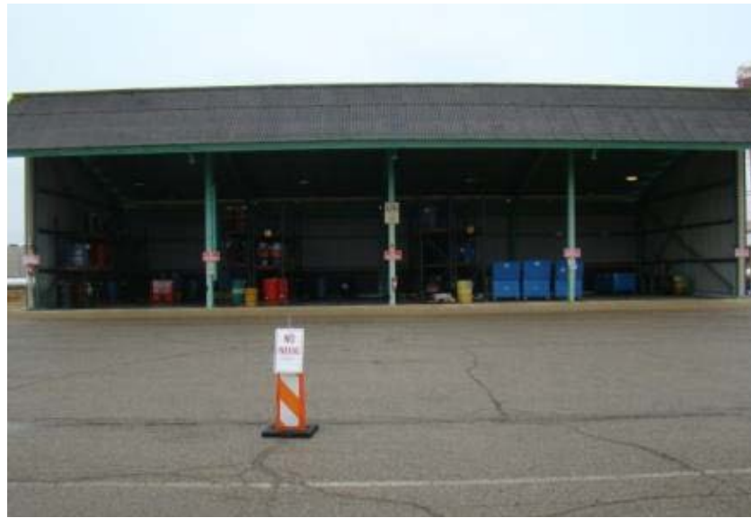
Figure A.121. X-741 Oil Drum Storage Facility
