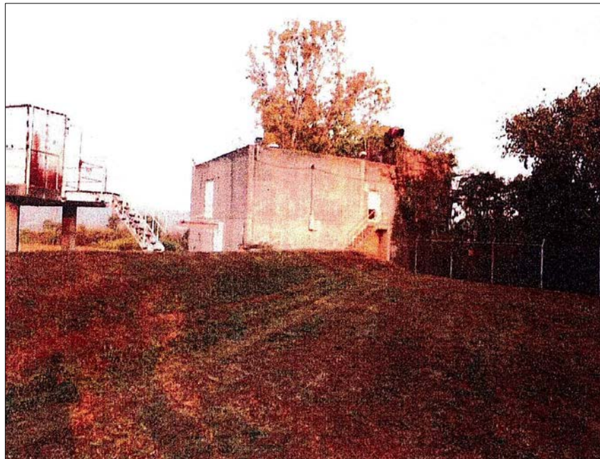
Figure A.80. X-608 Raw Water Pump House
