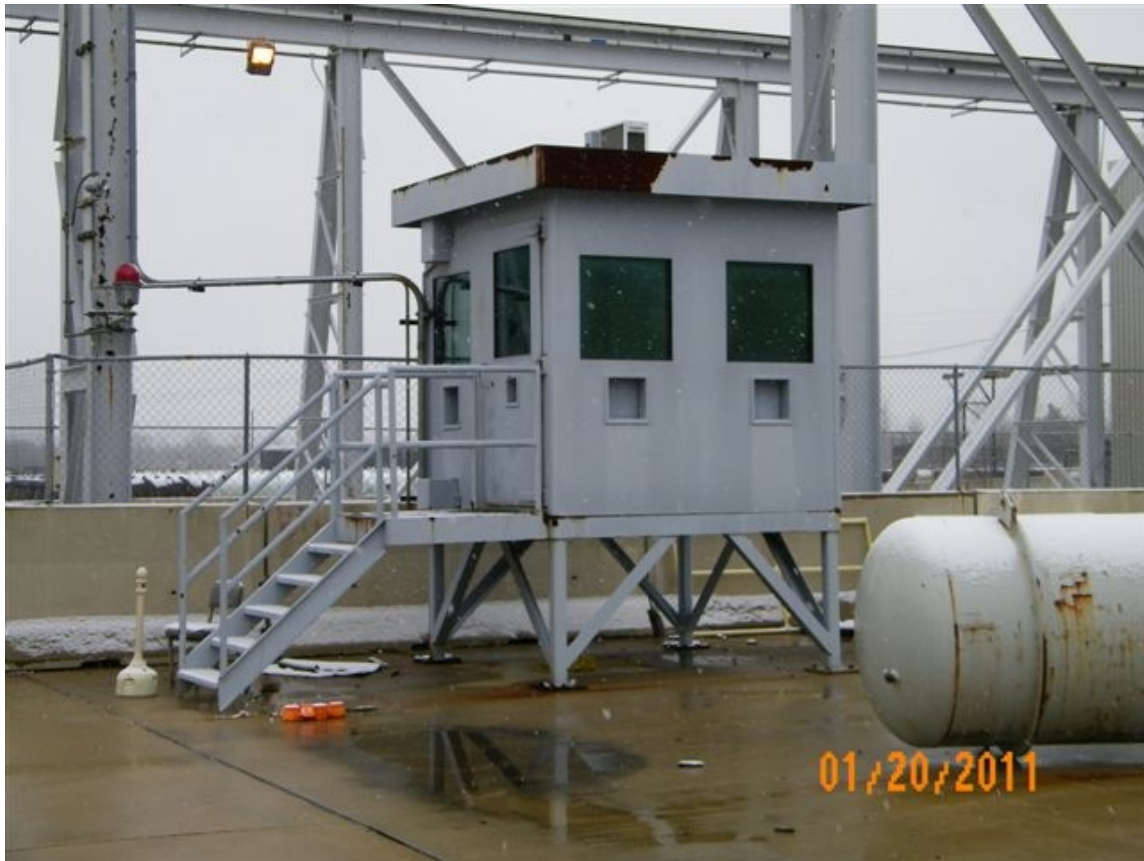
Figure A.52. X-344H Security Portal
