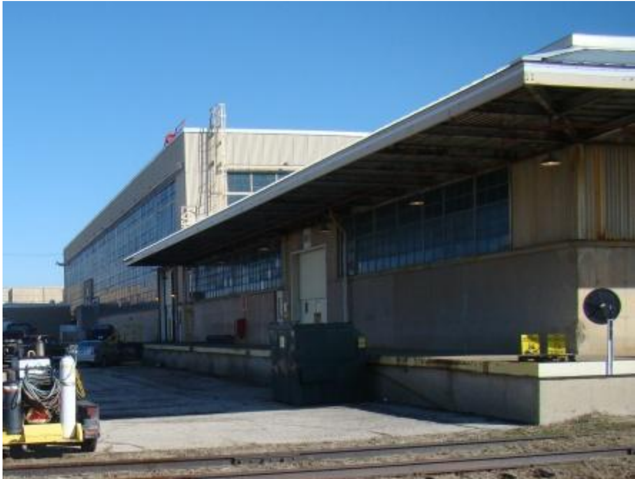
Figure A.36. X-720 Maintenance & Stores Building
