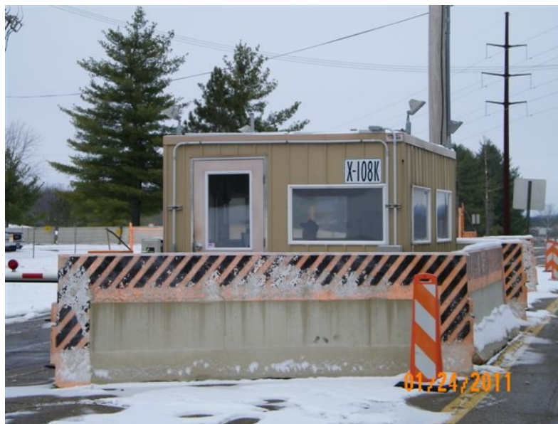
Figure A.48. X-108K North Security Portal
