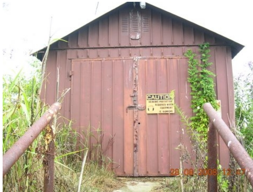
Figure A.78. X-605 Sanitary Water Control House Exterior
