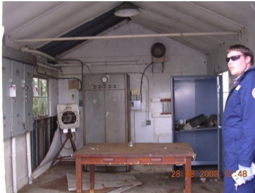
Figure A.79. X-605 Sanitary Water Control House Interior
