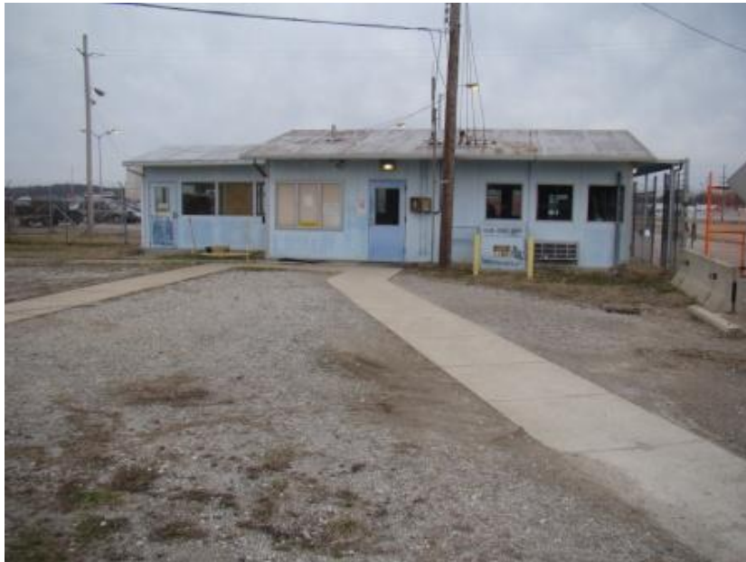
Figure A.46. X-108E Construction Entrance Portal
