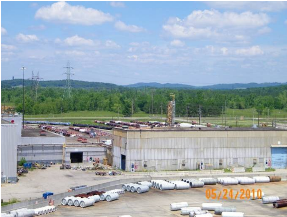
Figure A.16. X-342A Feed Vaporization Building
