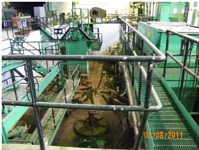
Figure A.38. X-720 Maintenance & Stores Building Shop Areas
