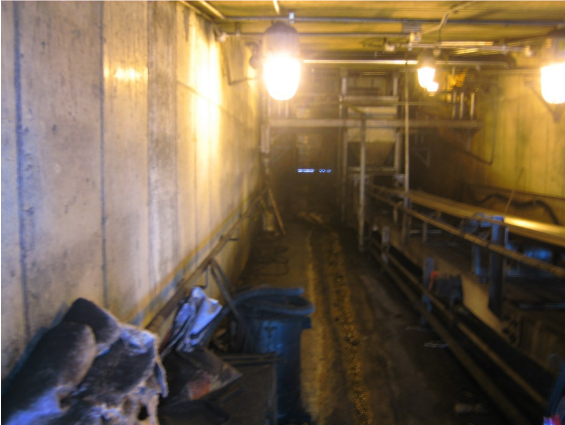
Figure A.114. X-600A Coal Belt Pit (below-grade structure)
