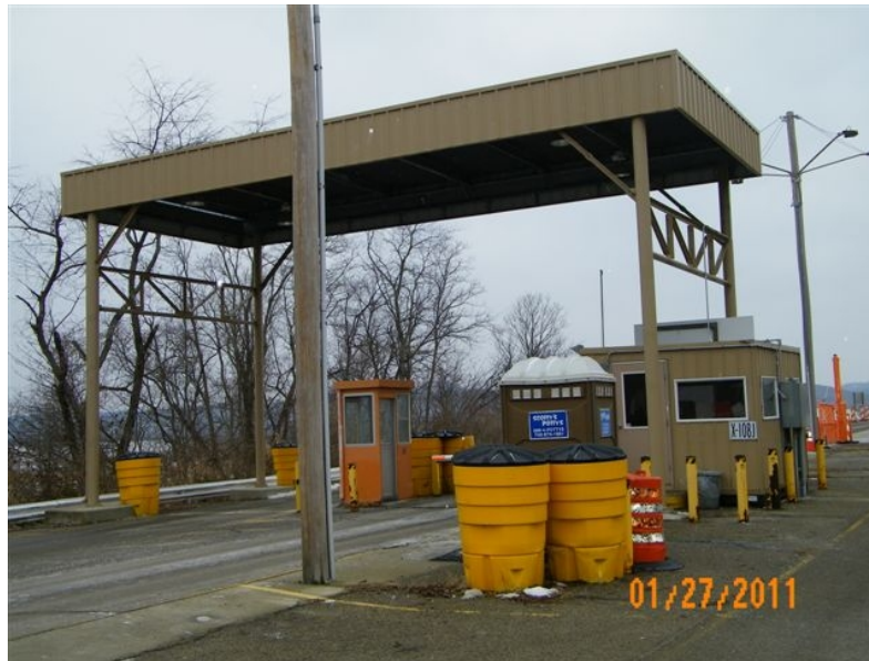
Figure A.47. X-108J West Security Portal
