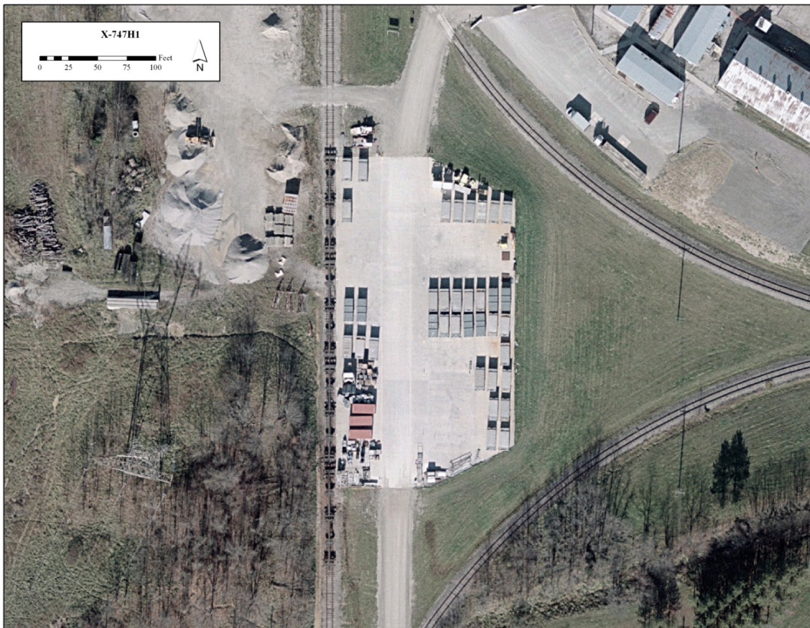
Figure A.145. X-747H1 Loading Pad (2006-2007 Aerial Photography)
