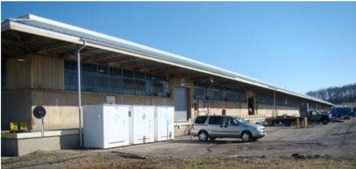
Figure 4.8. X-720 Maintenance & Stores Building at PORTS
