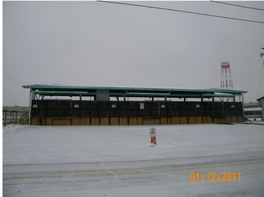
Figure A.124. X-742 Gas Cylinder Storage Facility
