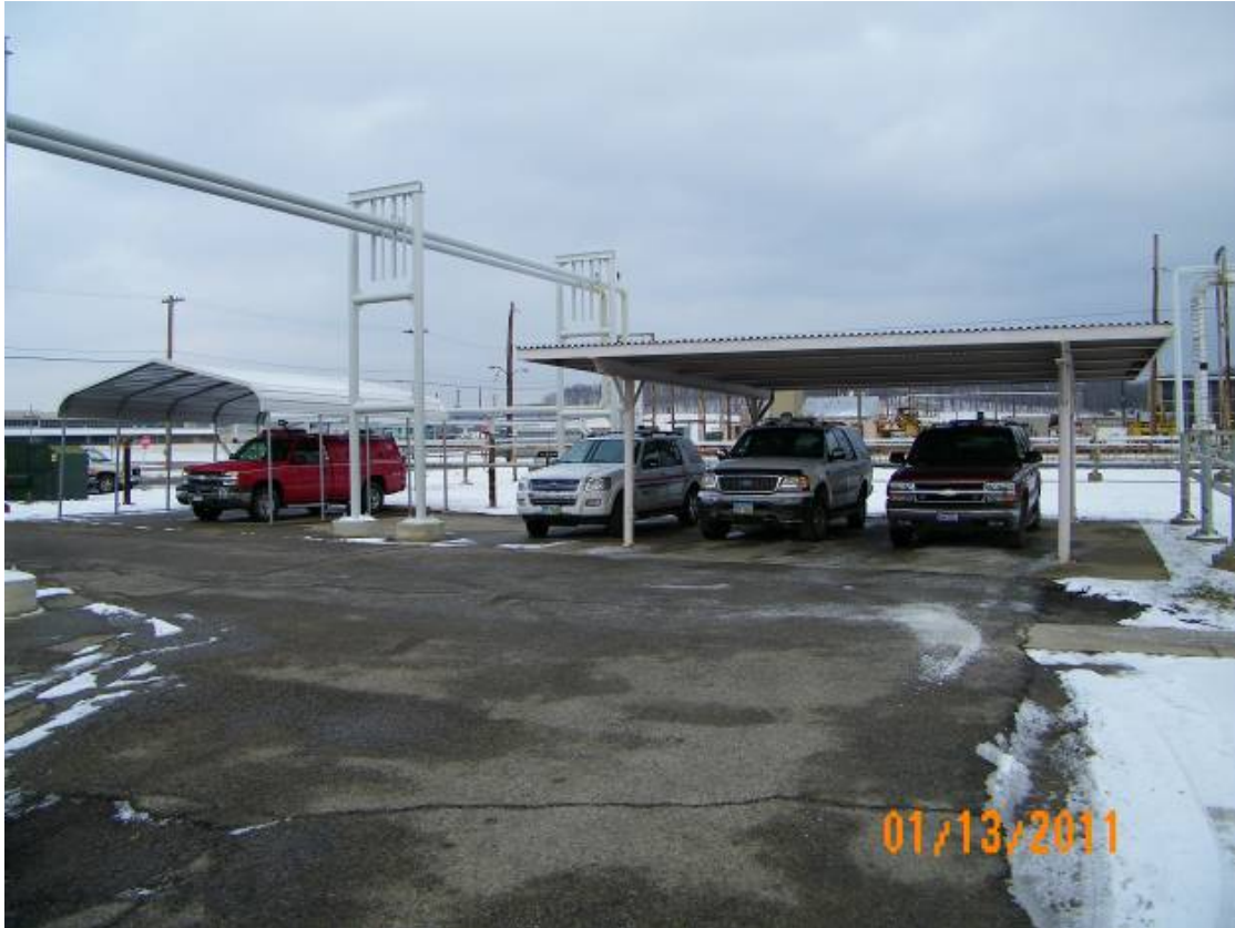
Figure A.61. X-300B Plant Control Facility Carport
