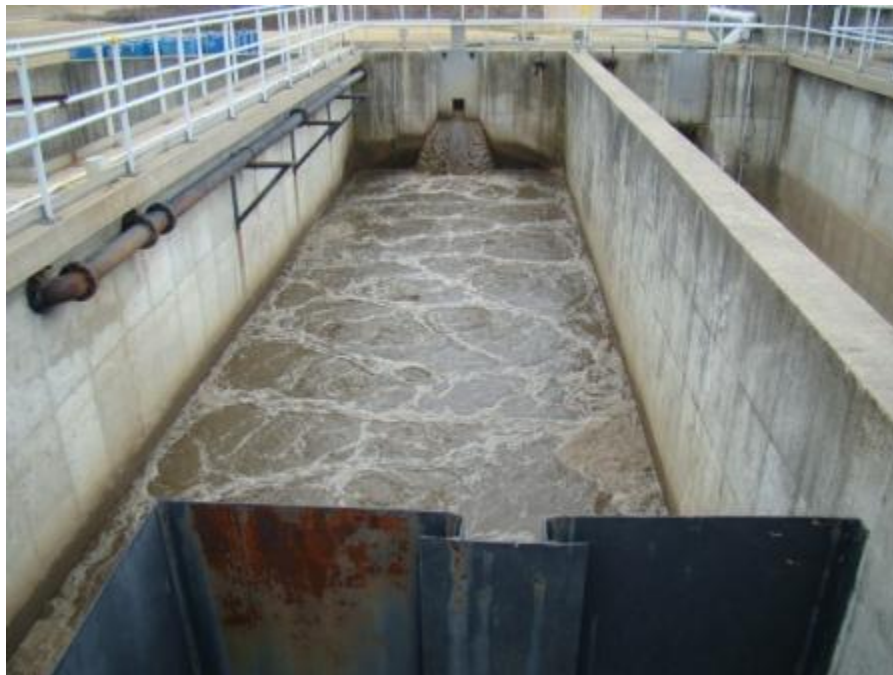
Figure A.100. X-6619 Sewage Treatment Plant, Aeration Tanks
