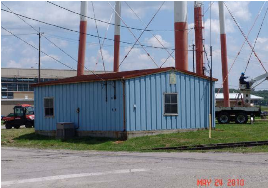
Figure A.40. X-720B Radio Base Station
