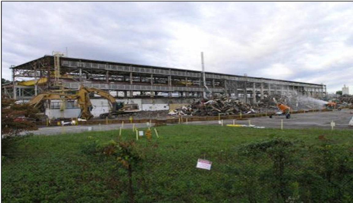
Figure 7.7. Example of Support Building Demolition at ETTP
