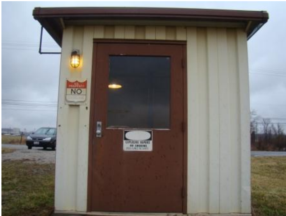
Figure A.89. X-614D South Sewage Lift Station
