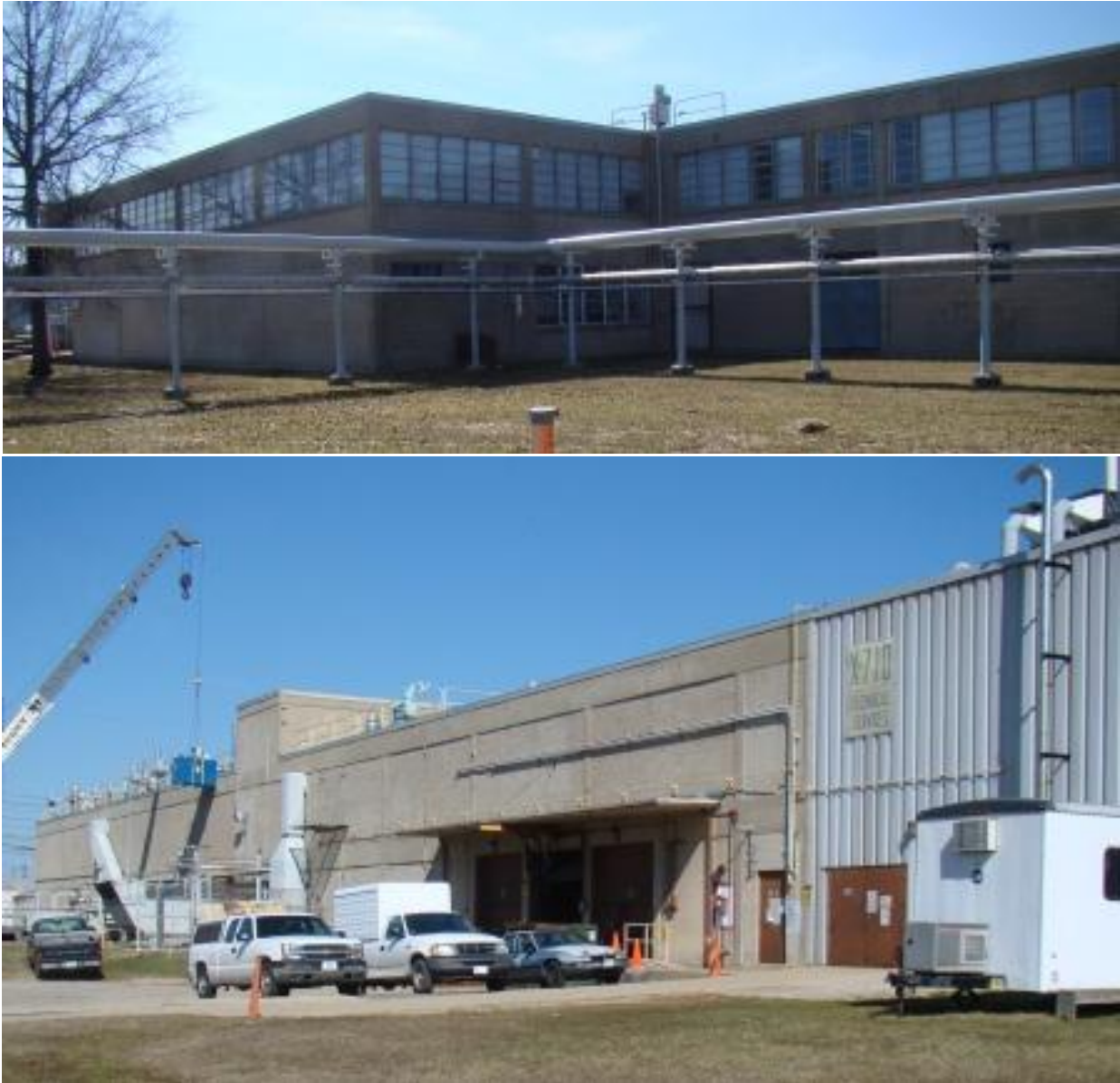
Figure A.31. X-710 Technical Service Building
