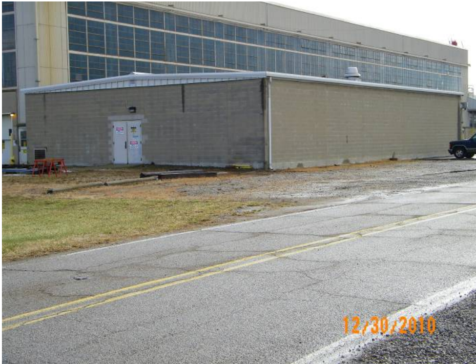
Figure A.42. X-720C Paint & Storage Building
