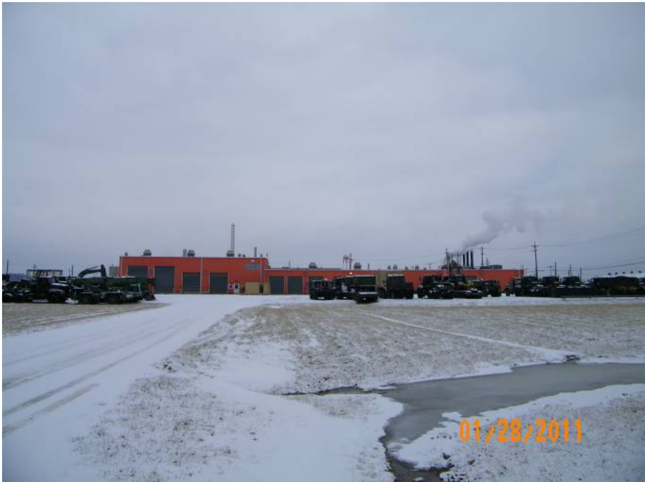
Figure A.67. X-751 Mobile Equipment Garage
