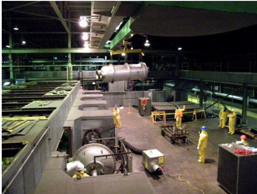
Figure 7.3. Movement of X-326 Converter
