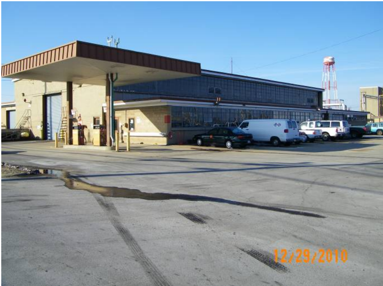
Figure A.66. X-750 Mobile Equipment Maintenance Shop
