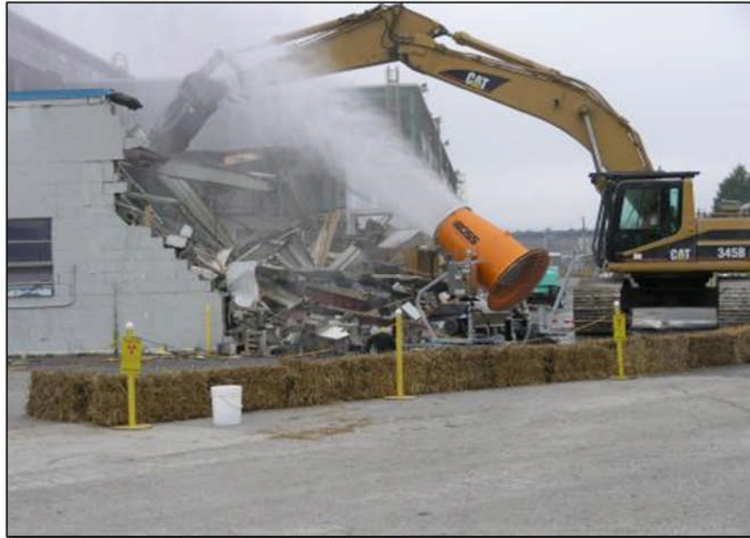
Figure 7.5. Example of Misting Technique
