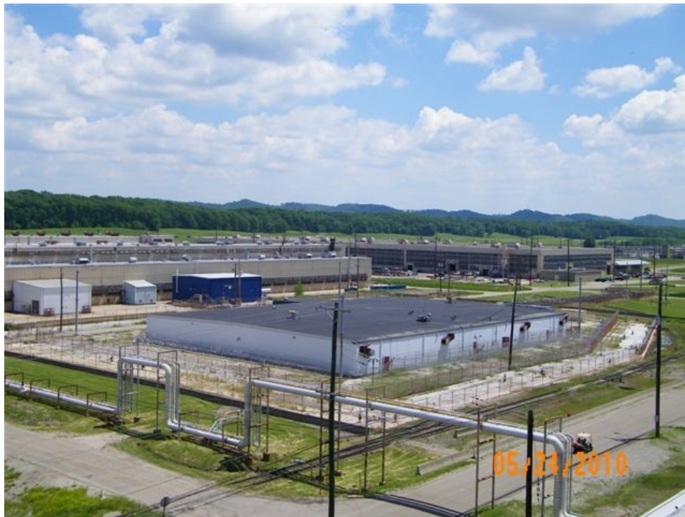
Figure A.118. X-345 SNM Storage Building
