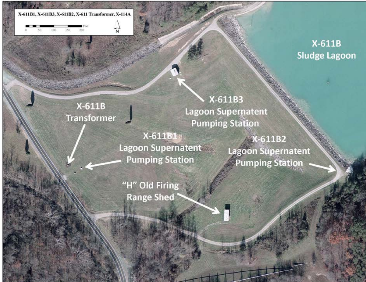
Figure A.85. X-611B Structures (2006-2007 Aerial Photography)
