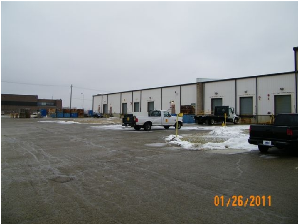
Figure A.147. XT-847 West Side Loading Docks and Parking
