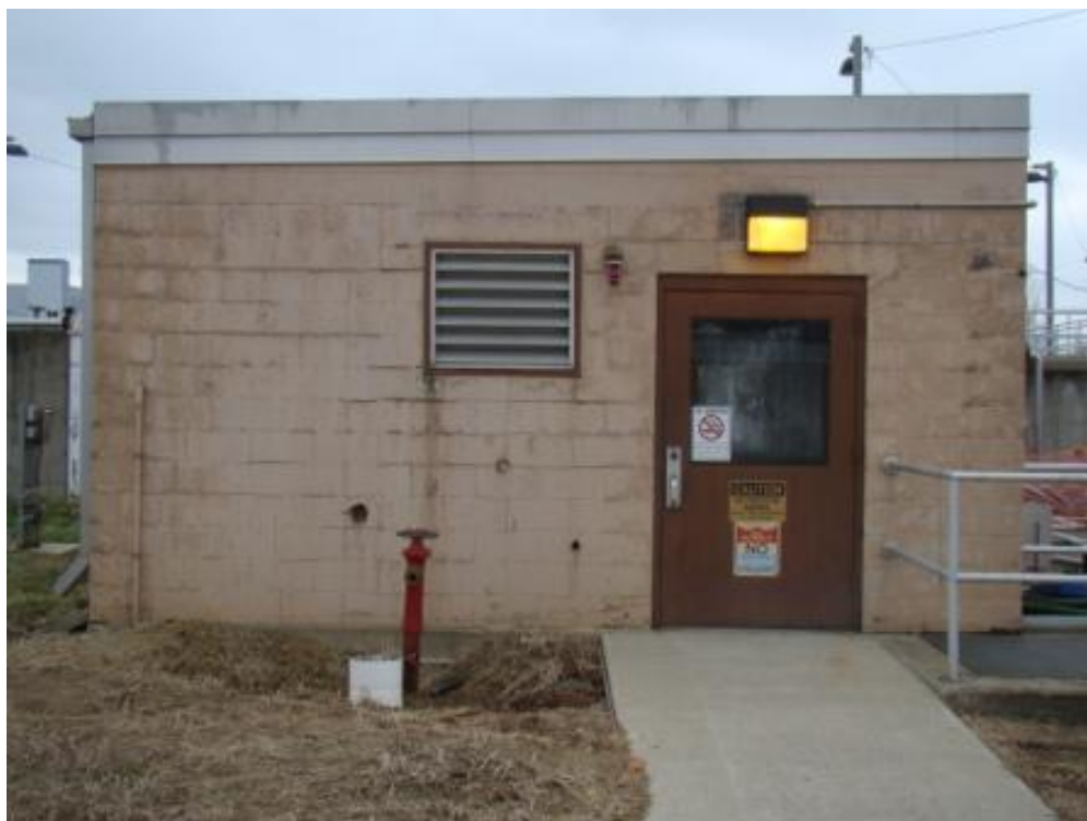
Figure A.98. X-6619 Sewage Treatment Plant, Sludge Pumping Building
