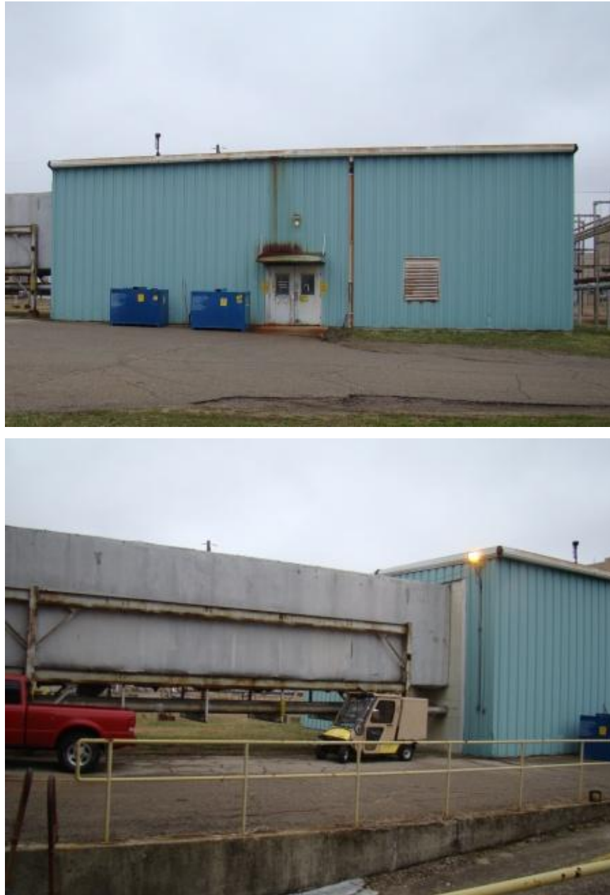
Figure A.22. X-700A Air Conditioning Equipment Building
