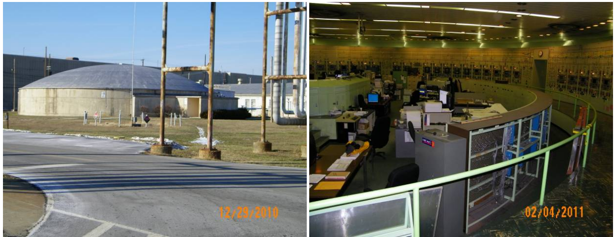
Figure A.58. X-300 Plant Control Facility
