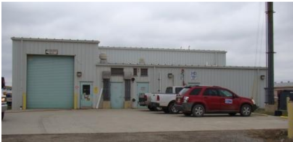
Figure A.177. X-623 North Groundwater Treatment Building
